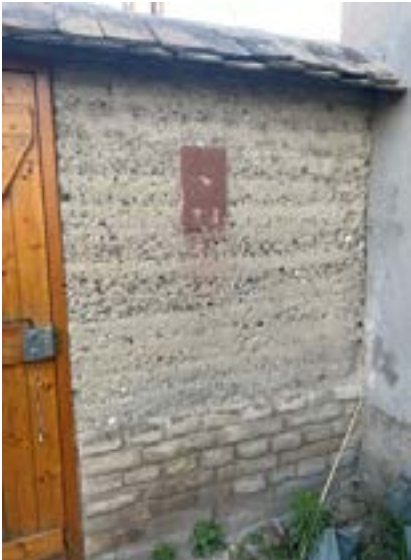
Zid iz zbite zemljine Wall made from rammed earth
